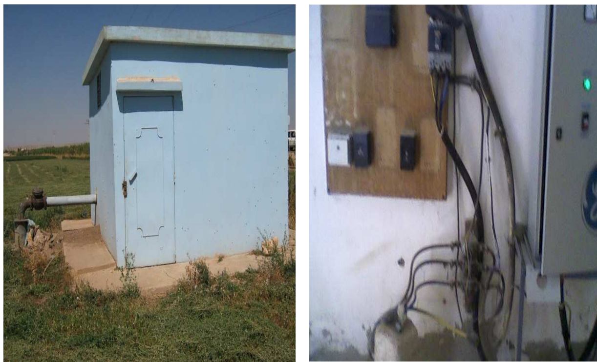
Figure II-2: Vue du forage CH3.
