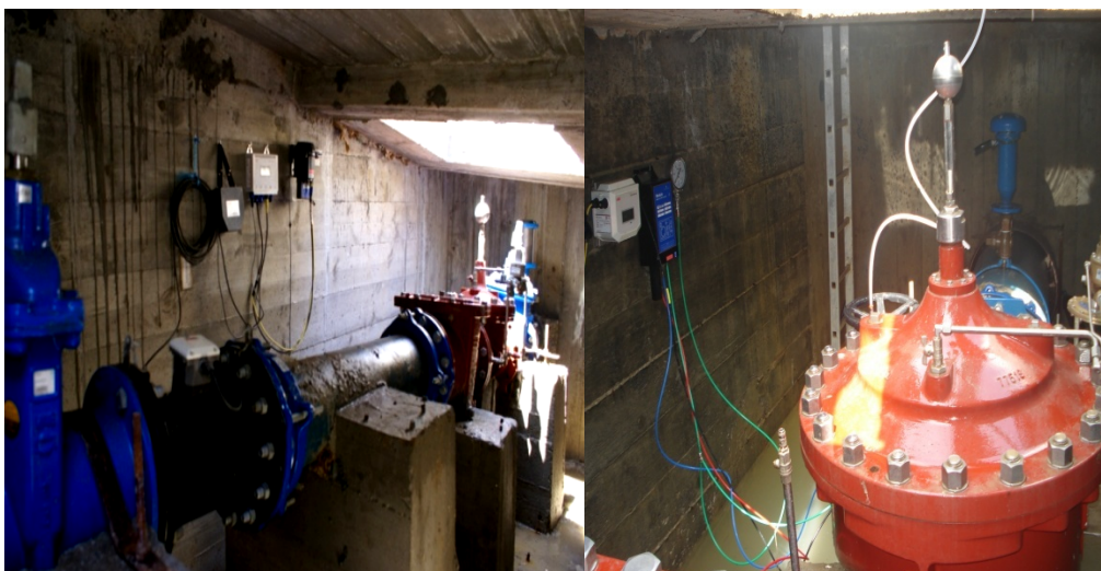
Figure III.15: Vanne de modulation Kouba117. [Document technique. SEAAL.2010].
