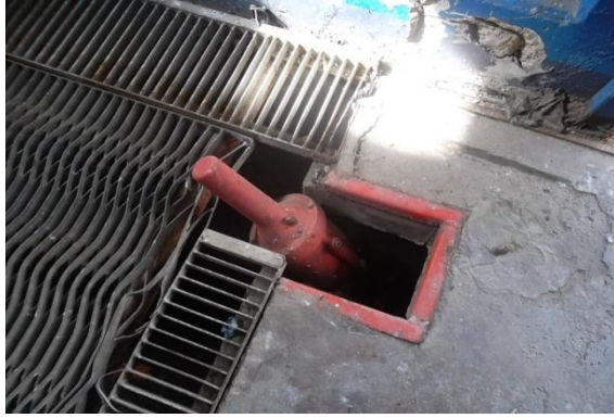
Figure III-6 : Clapet anti –choc
