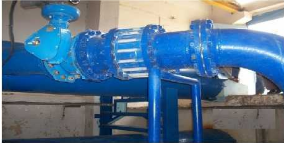
FigureV.5: Joint, Coude et clapet anti-retour
