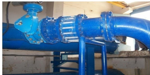
Figure V-10 : Joint, Coude et clapet anti-retour.
