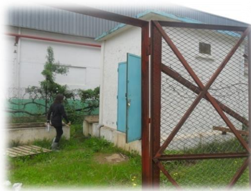
Figure 5 : Photo du forage SAIDAL
