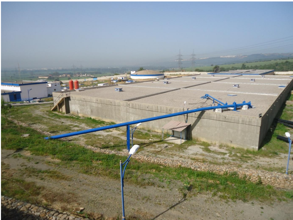
Figure II.1 :Le complexe hydraulique SP3.
