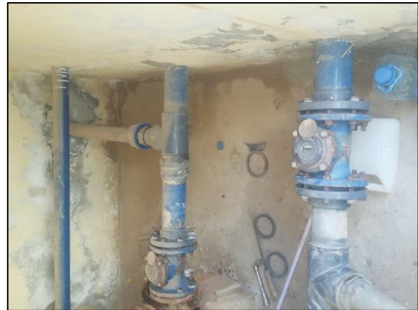
Figure III.31 : Les vannes de distribution R100.
