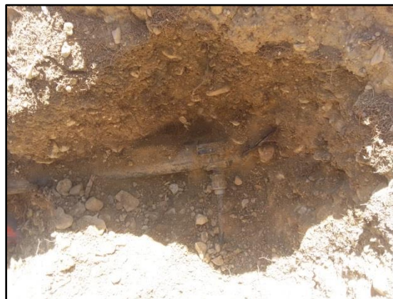
Figure III.23 : Branchement de distribution R50.
