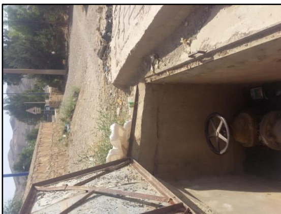
Figure III.34 : Vannes de distribution N55.
