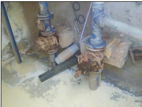
Figure III.31 : Les vannes de distribution R100.
