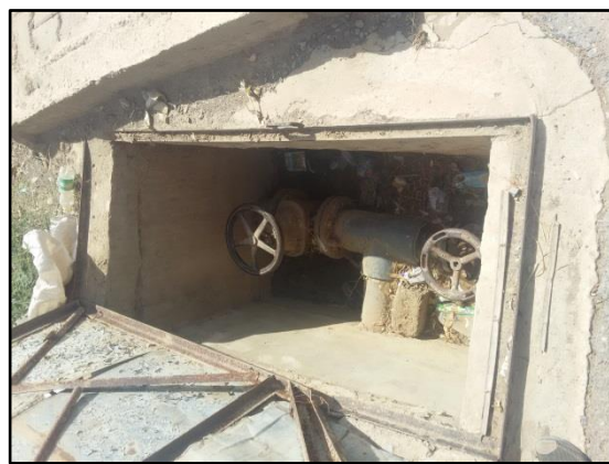
Figure III.34 : Vannes de distribution N55.
