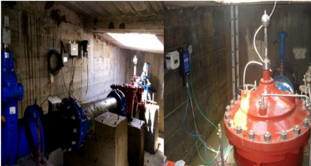
Figure III.20 : vanne de modulation ( Kouba ,97)
