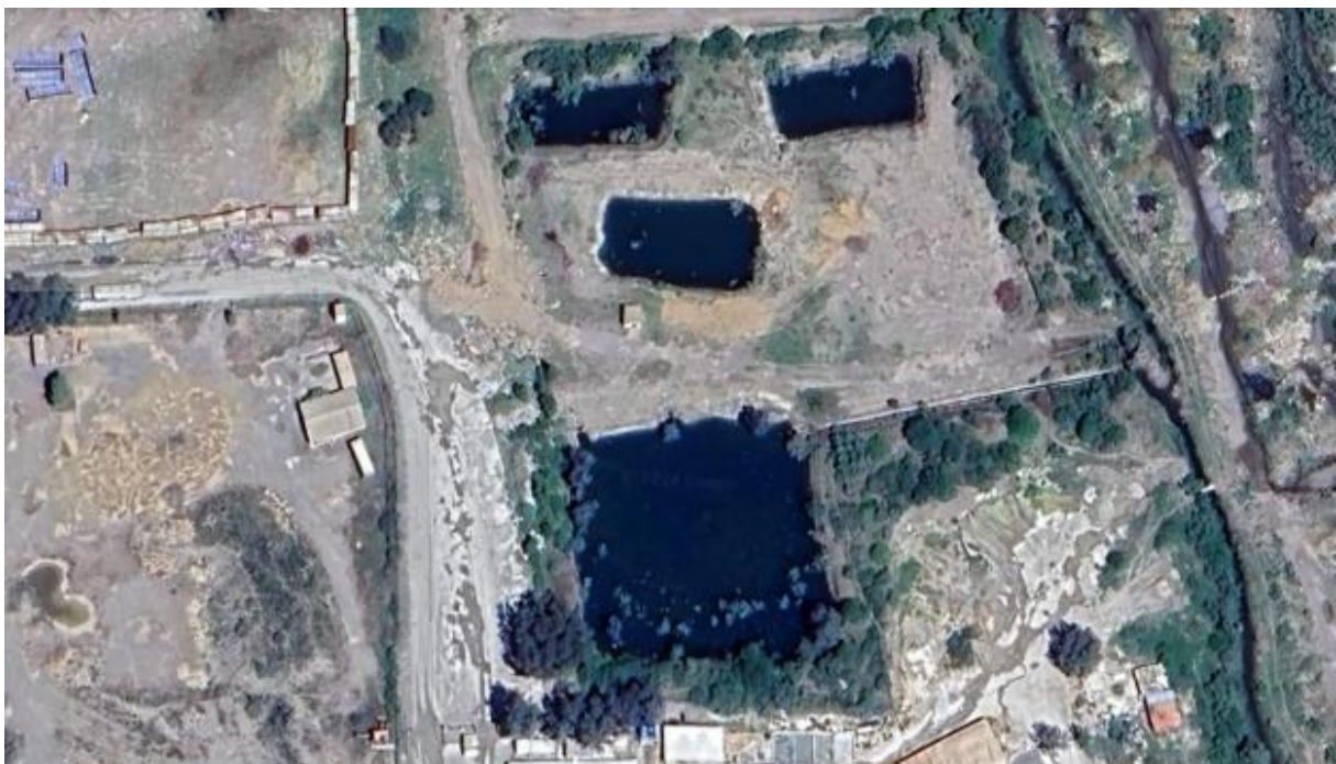
Figure II.5 : Bassins d'infiltration (Google Earth,2024)
