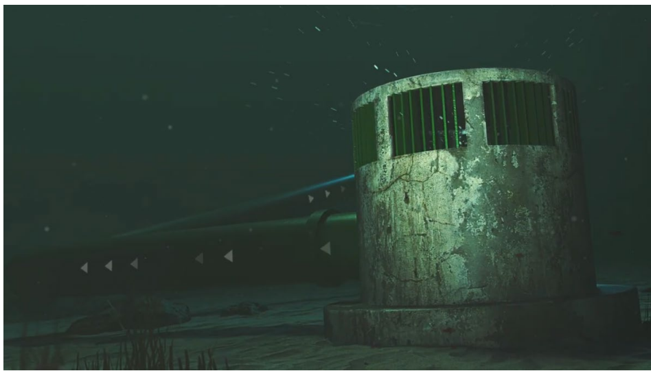
Figure 11: La tour de captage
