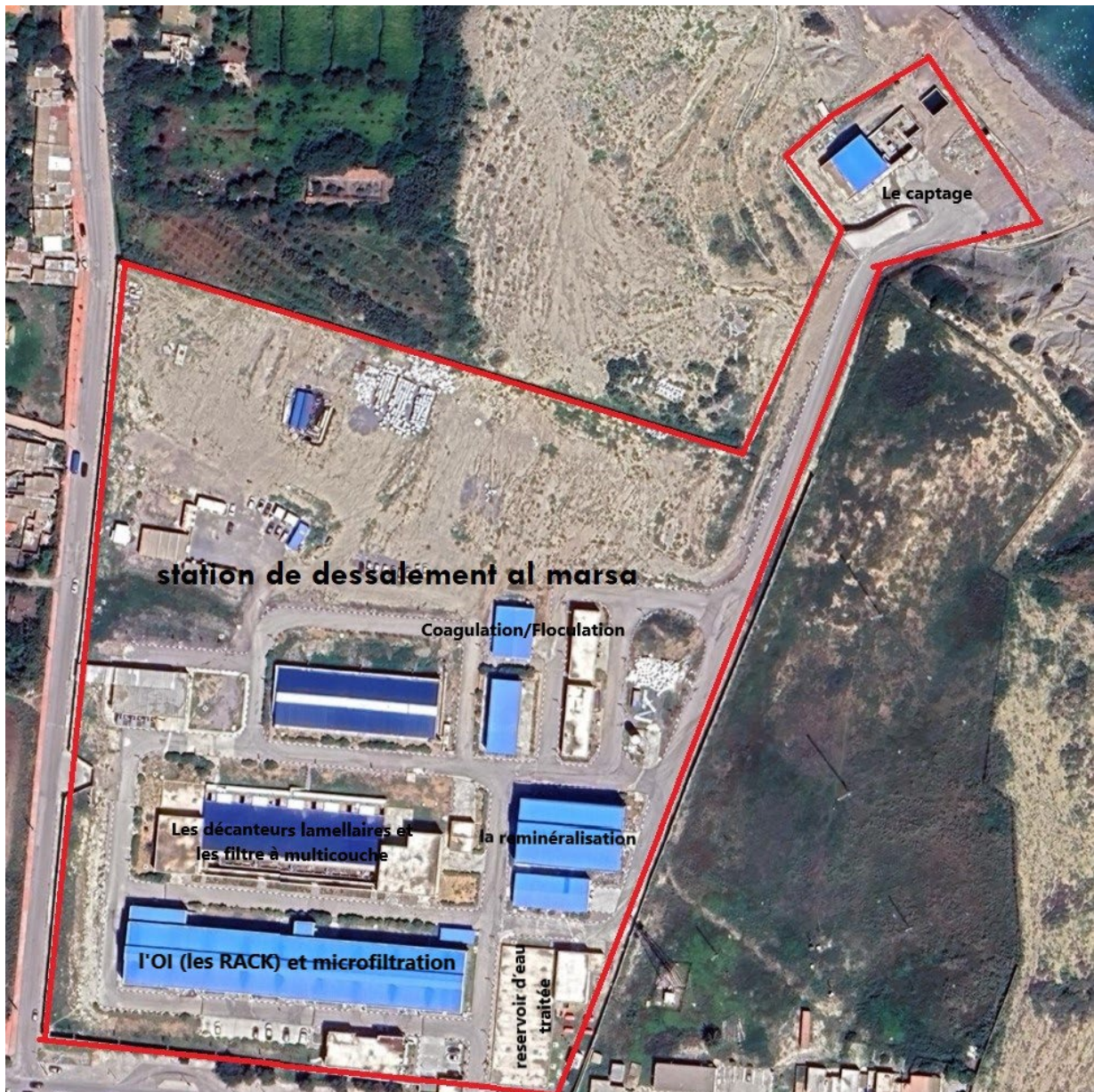
Figure 10: la station de dessalement El Marsa
