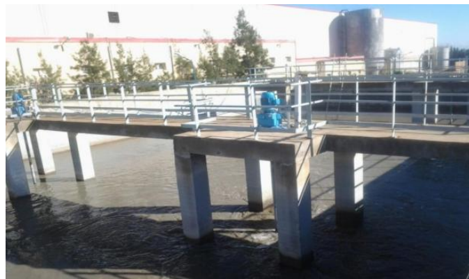
Figure I.4 Bassin homogenization de STEP Tonic
