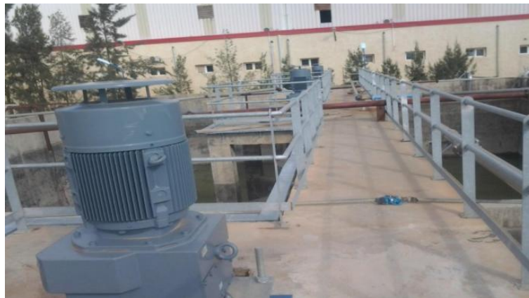
Figure I.9 Bassin aeration de STEP Tonic
