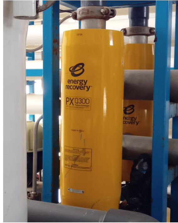
Figure III.16 : ER pressure exchanger
