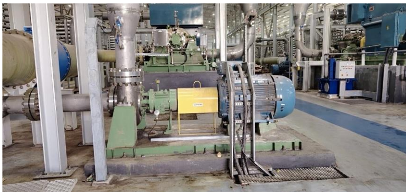
Figure III. 10 : pompe booster
