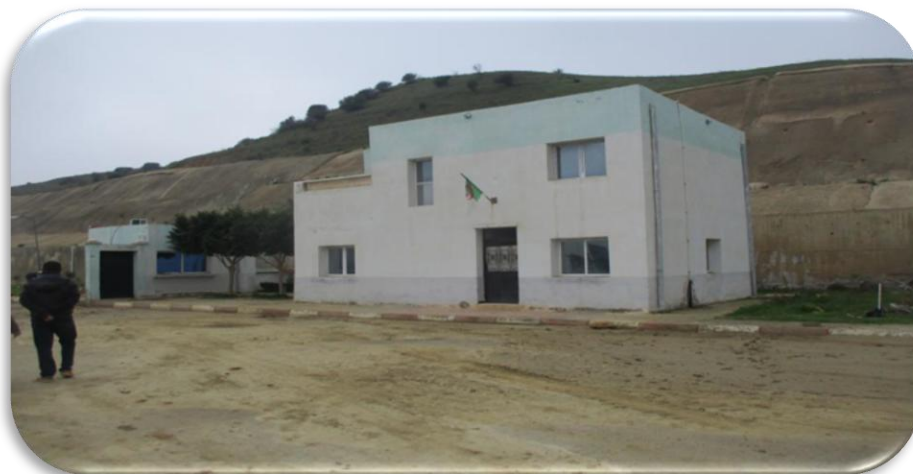
Figure III.5 : Station de relevage
