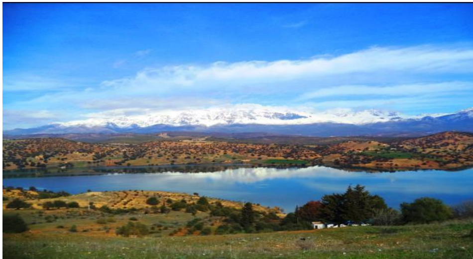
Figure III-2: Barrage de TILES DIT.
