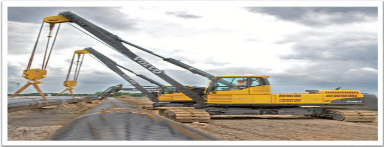
Figure (VII-7) : le pipelayers.
