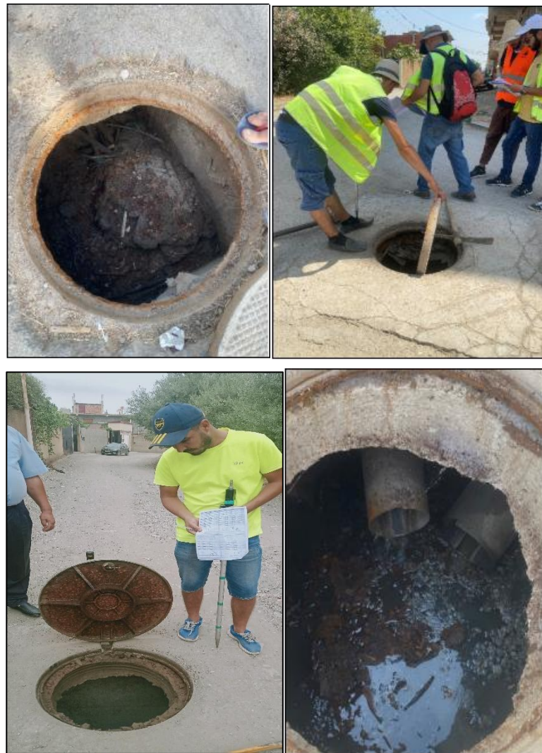
Figure III.3: Etat des regards
