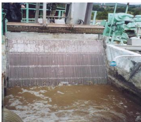
Figure III-3 : Grille manuelle
