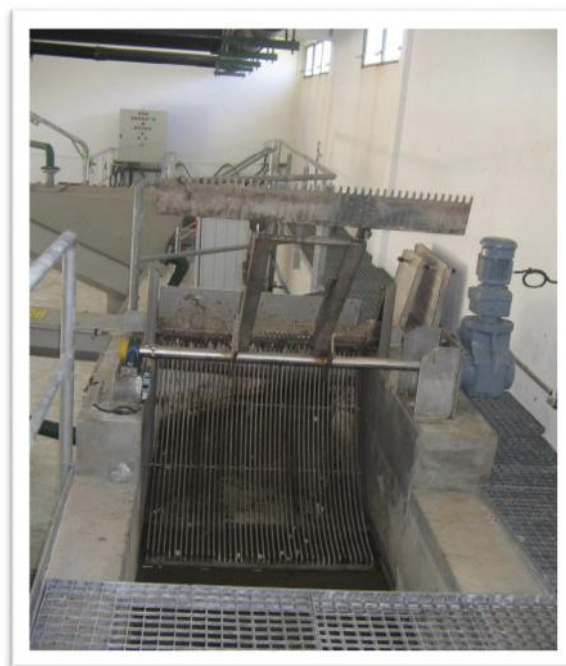
Figure III.4: grille mécanique
