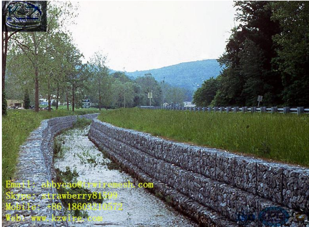
Figure III.9 : canal en gabion
