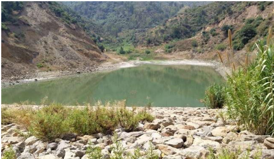
figure I-2 : Retenue Oued El Had
