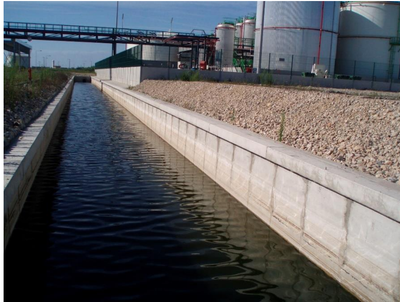
figure III-3: Canal en Béton (source :Google)
