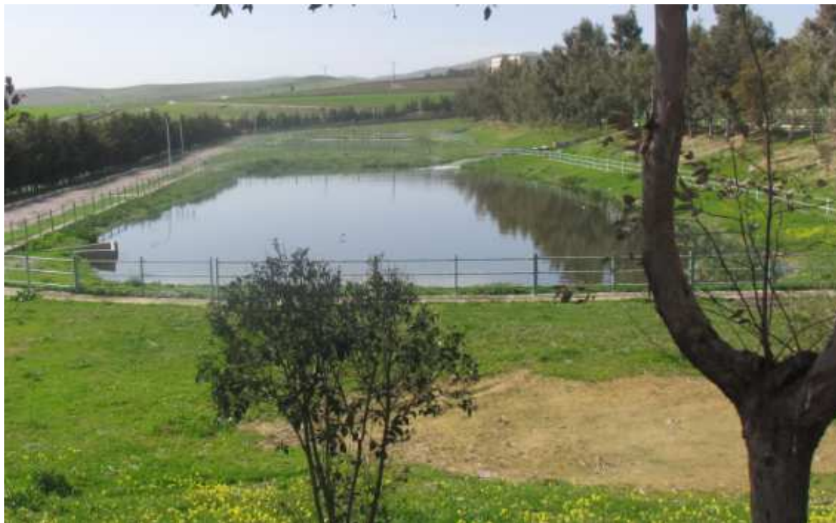
Figure III.5: Bassin de maturation
