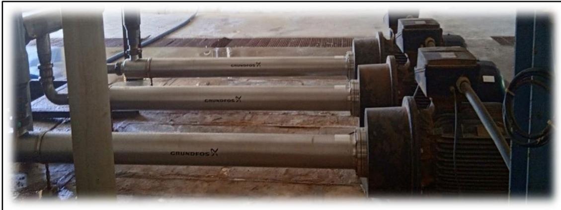
FIGURE IV.34 : POMPE A HAUTE PRESSION.
