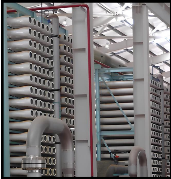
Figure II.8: Racks d'osmose inverse (L'installation de SOUK THLATHA)
