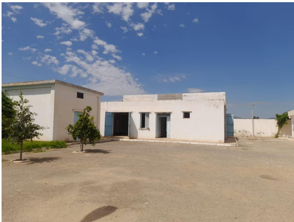
Figure I. 3: station de pompage (14/05/2024).
