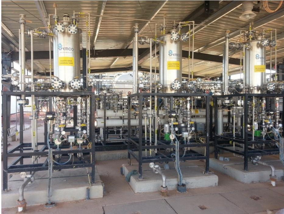
Figure IV.3: Chemical feed system (2 may 2024, GRN)
