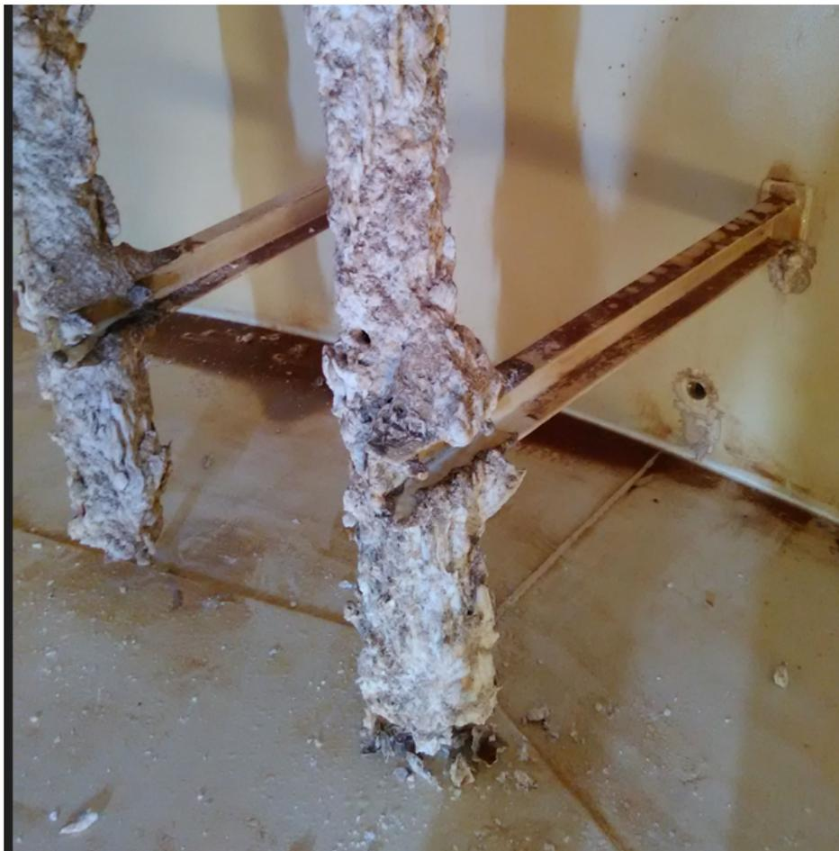
Figure IV.11: Picture of depositions inside the raw water tank during the last cleaning (2022)
