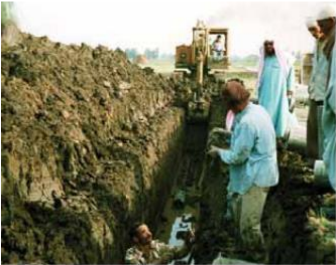
Figure IV.6: Hydraulic excavator digging a drain trench.
