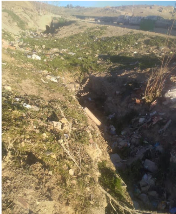
FIGURE 3.6 – Obstruction du canal
