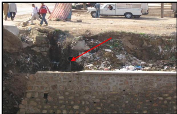
**Figure I.4 :** Rejet I DN 300 (Pont).
