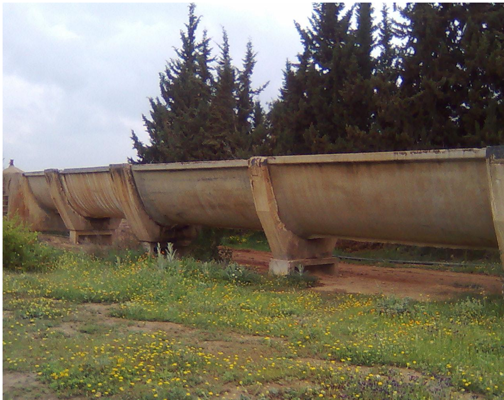
Figure 3 : Canal principal autoporté
