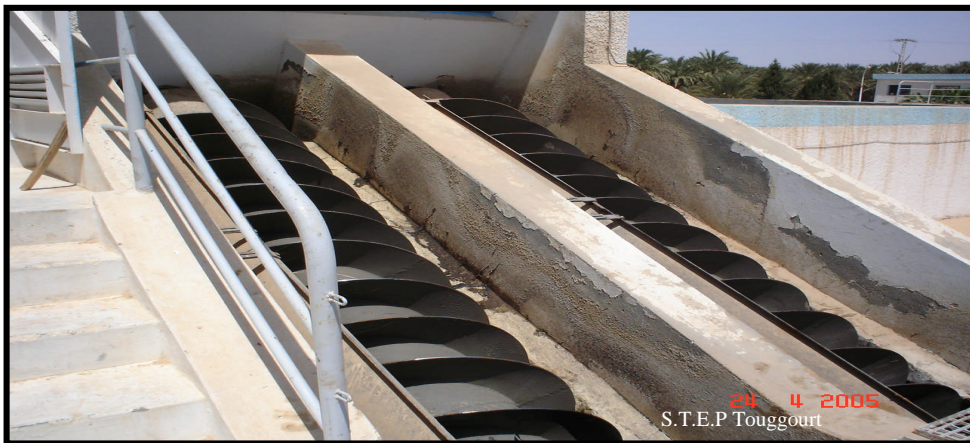
Figure IV-07: Vis Archimède
