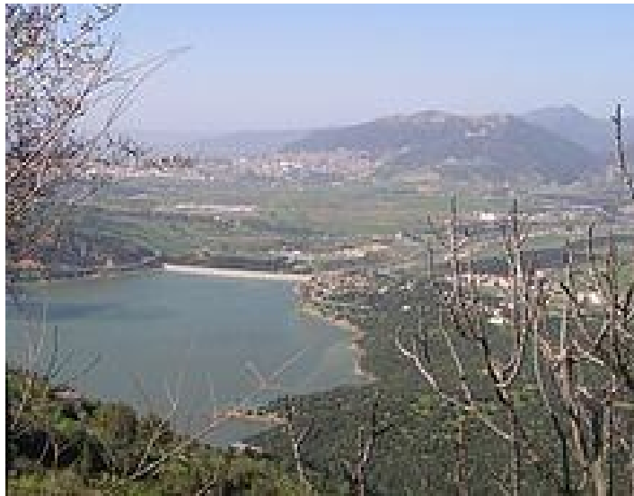
Figure II.4 : barrage de Tilesdit
