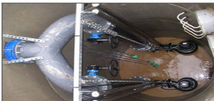
**Figure IV 38.** Station de relevage
