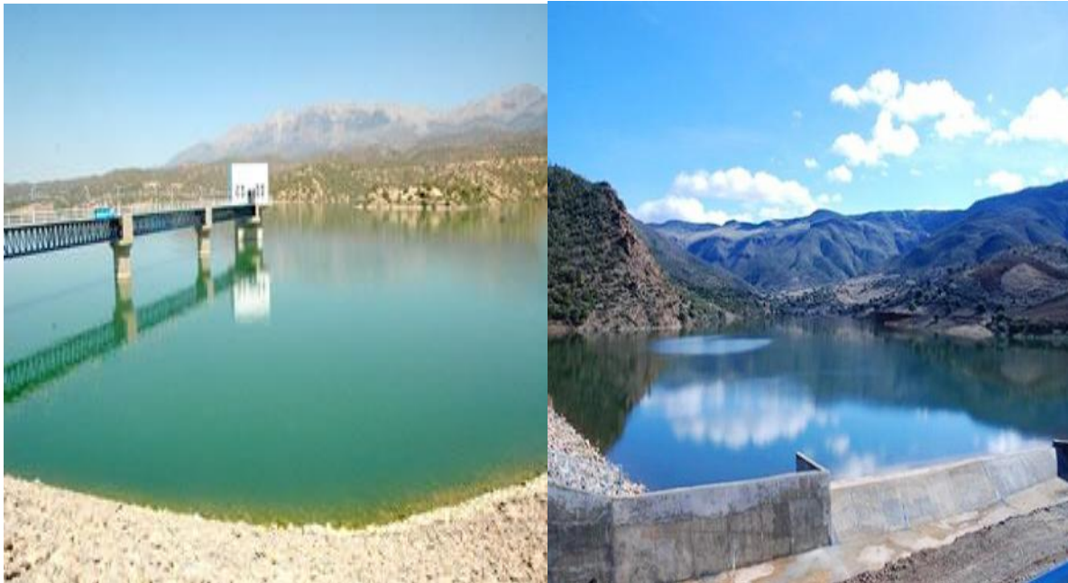
Figure II.2 barrage de Tilesdit
