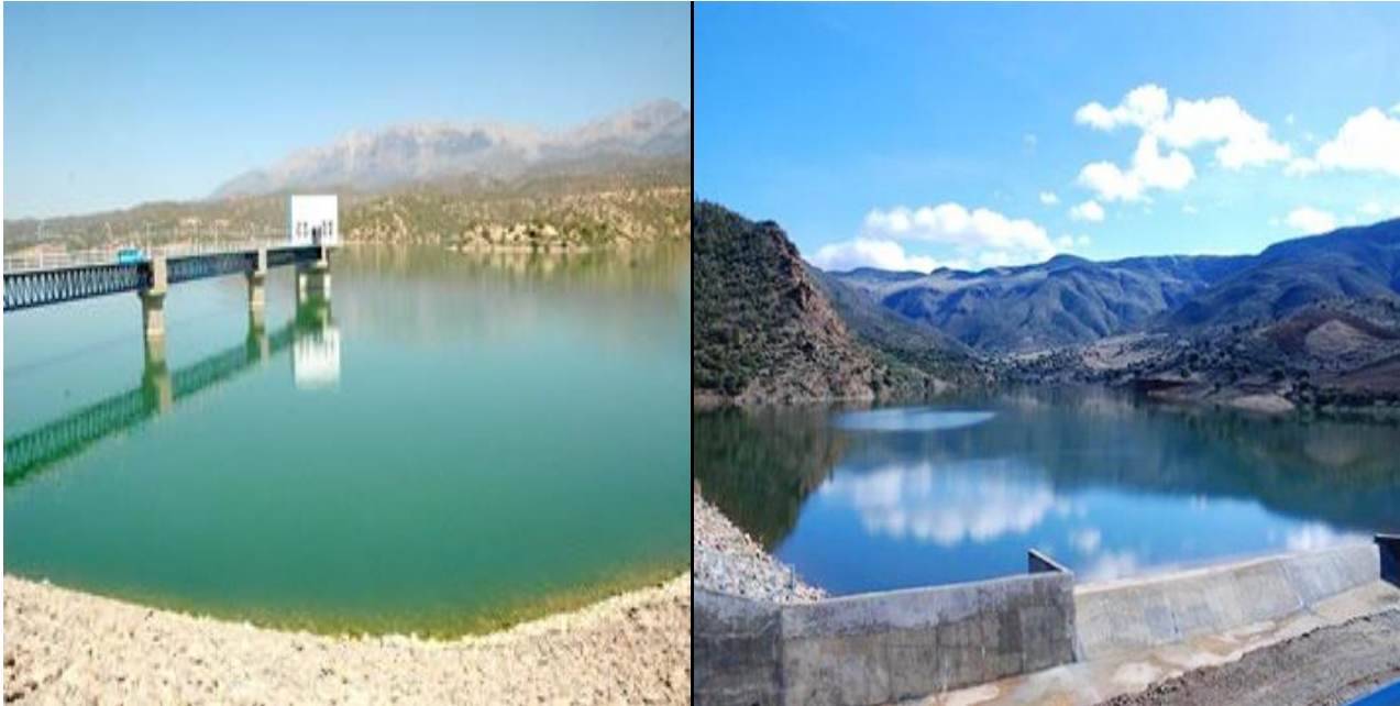
Figure II.2 barrage de Tilesdit
