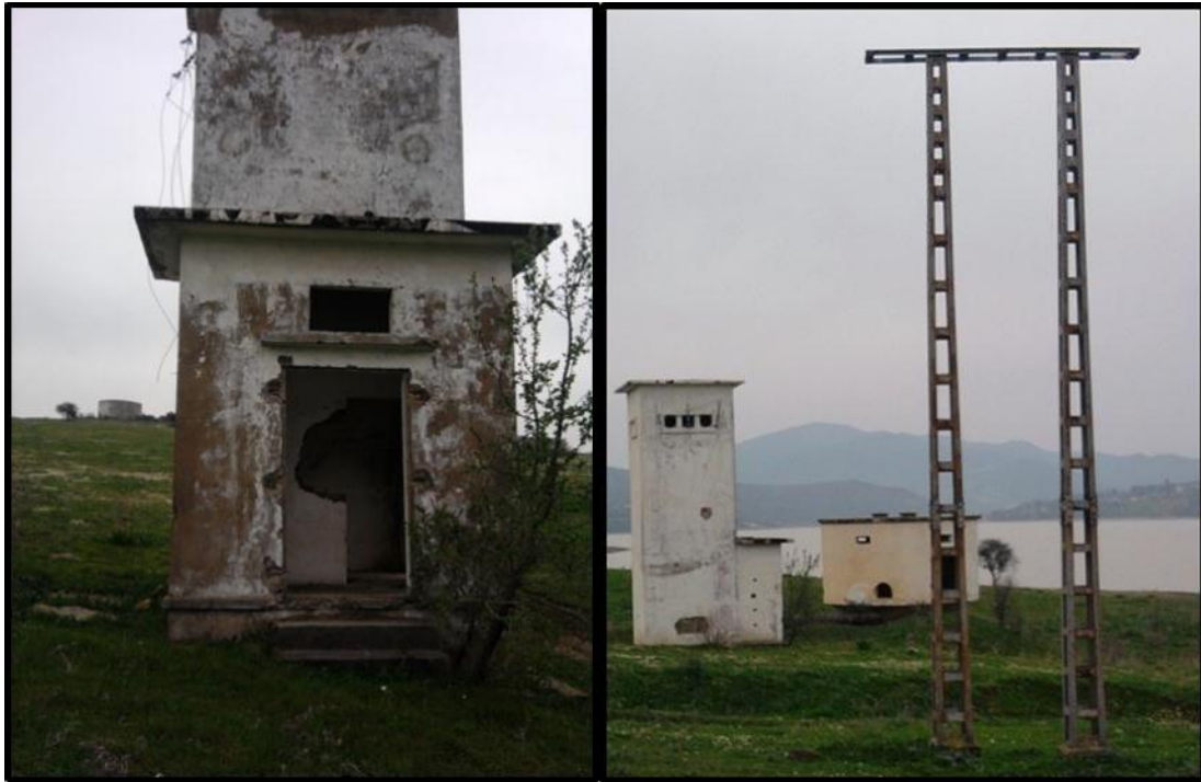
Figure IV -3: Station De Pompage
