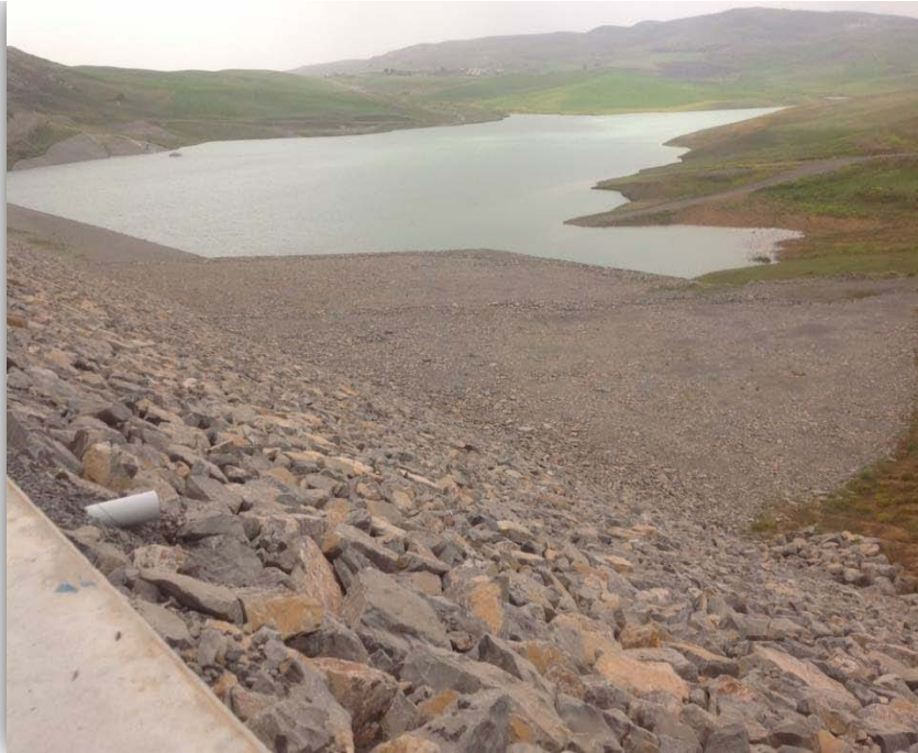
Figure III. 1: Barrage de MAHOUANE.
