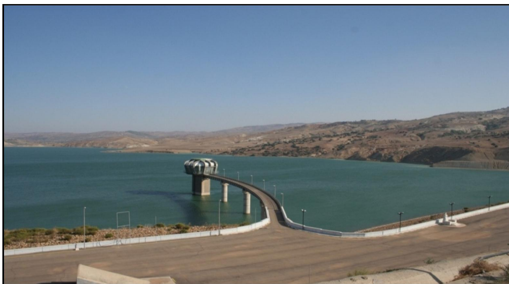
Figure III.2: Photo de barrage de Kramis (Source DRE.Mostaganem)
