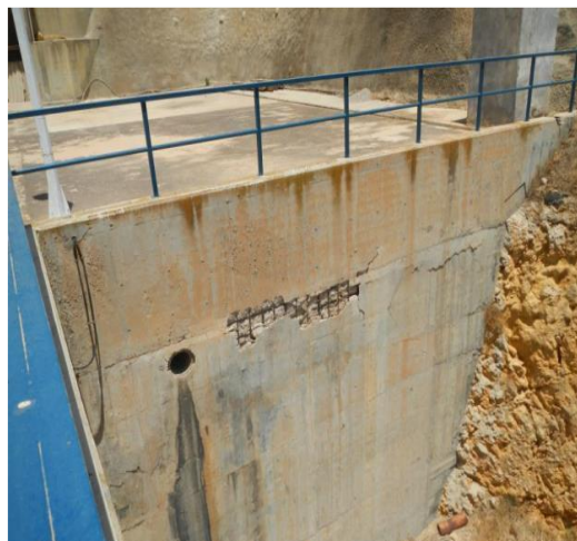
Figure III.6: Ferrailage apparent (appui rive gauche)
