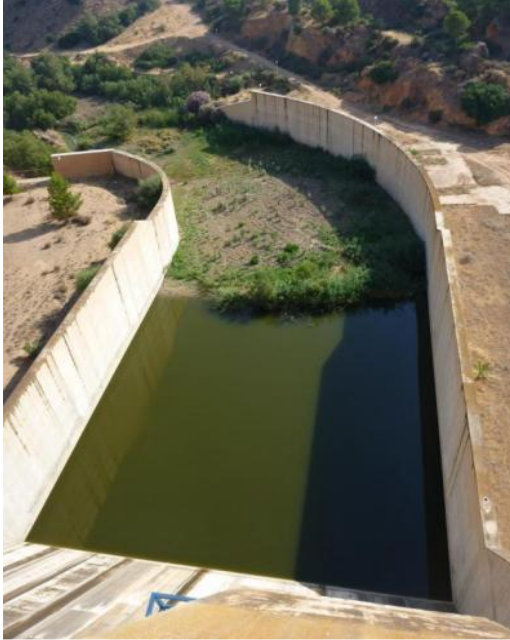
Figure III.31: Bassin dissipateur
