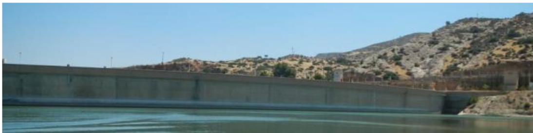
Figure III.2: Parement amont rive droite
