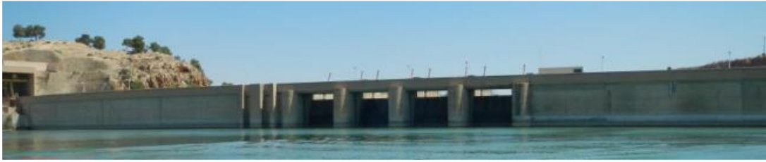
Figure III.1: Parement amont rive gauche
