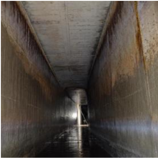
Figure III.37: Galerie de restitution enterrée
