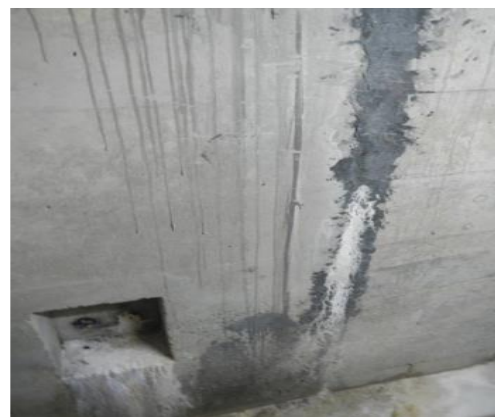
Figure III.19: Coulée de calcite sèche
