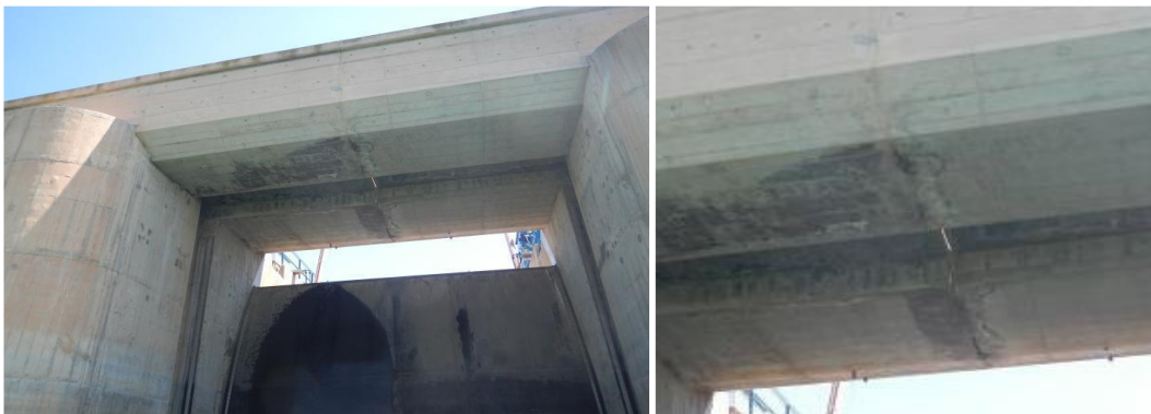
Figure III.27: Surface de la passerelle PH2 - PH3
