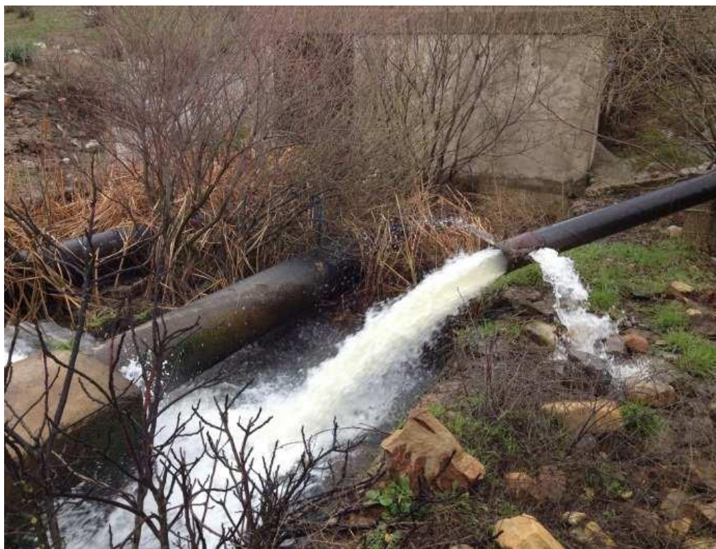
Figure II.26: Piquage DN 200 mm (ISL, 2015)
