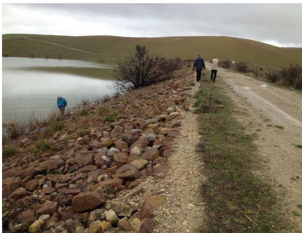
Figure II.4 : Bordure amont (ISL, 2015)
