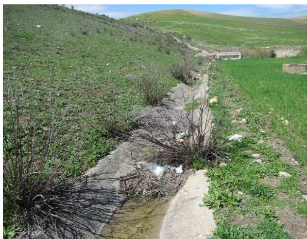
Figure II.6: Caniveau pied de talus (ISL, 2015)
