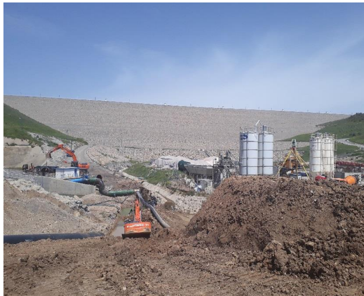
Figure III. 1: Barrage de MAHOUANE
