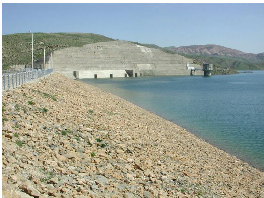
Figure II. 3. Photo du barrage d'Oued El-Athmania
