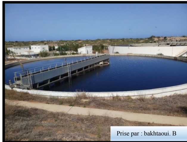
Figure III- 18 : Ouvrage de clarification.
