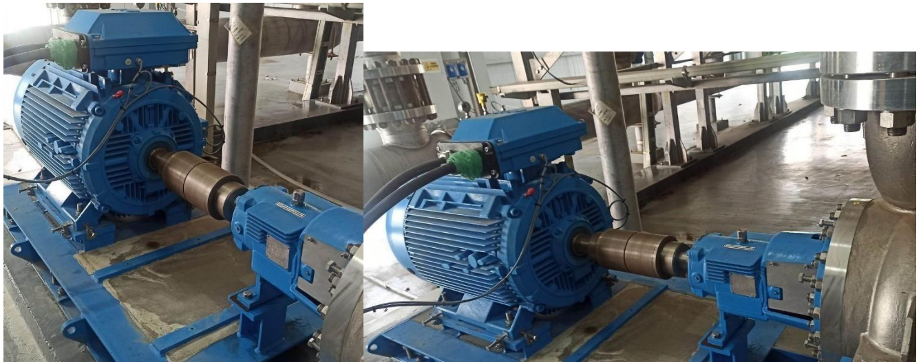
Figure IV- 16 Pompe Booster
