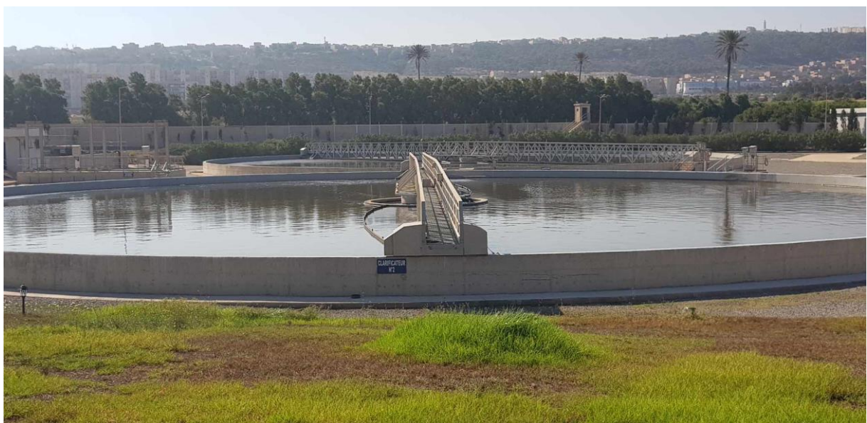
Figure III.12 : Clarificateur
