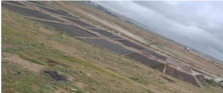
Figure III. 21: Lits de séchage.
