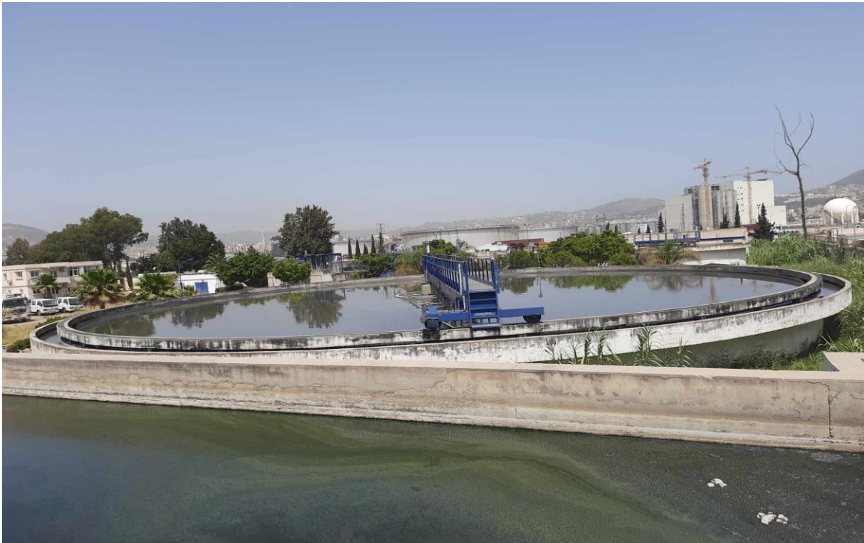
Figure 9: Clarificateur
