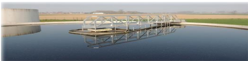
Figure.I.03: clarificateur
