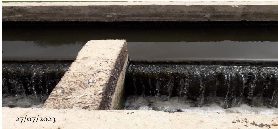
Figure IV.6 : Puit de coagulation.
