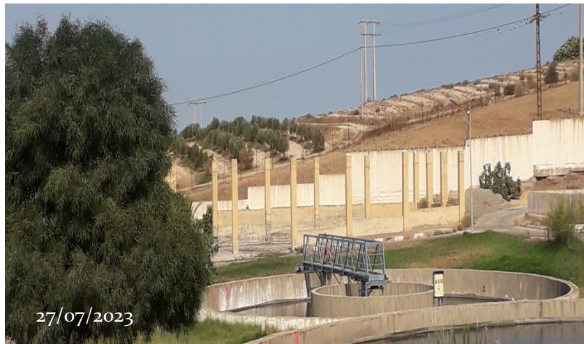
Figure IV.7: Clariflocculateur.
