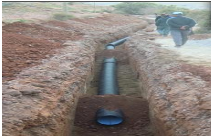
Figure 26 pose de canalisation.
